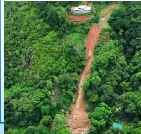
Photo: Drone shot capturing the landslide damage at Bel Ombre caused by heavy rains.
